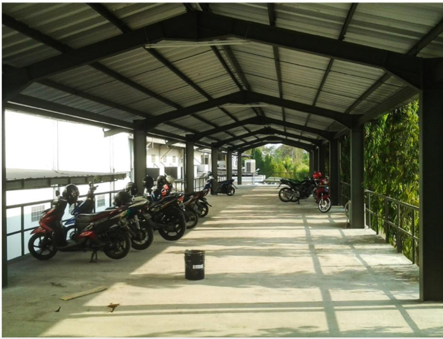
PT. Cahaya Jakarta Parking Building Cikarang, Jawa barat (2015)
